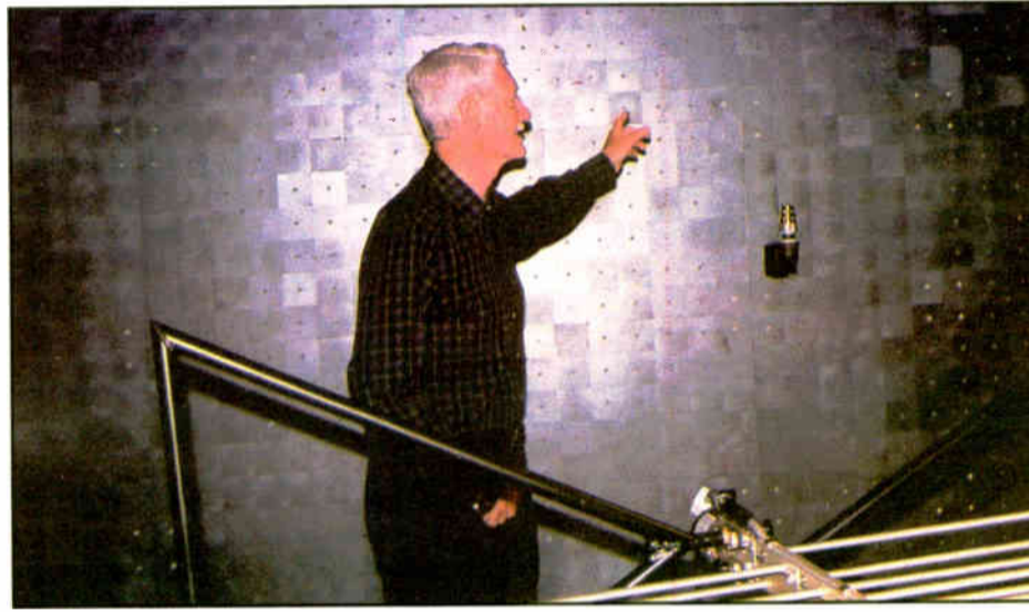
Engineer Tom Phillips displays ferrite tiles on the wall of the anechoic chamber. The tiles and carbon-impregnated foam, not shown, absorb higher frequencies
