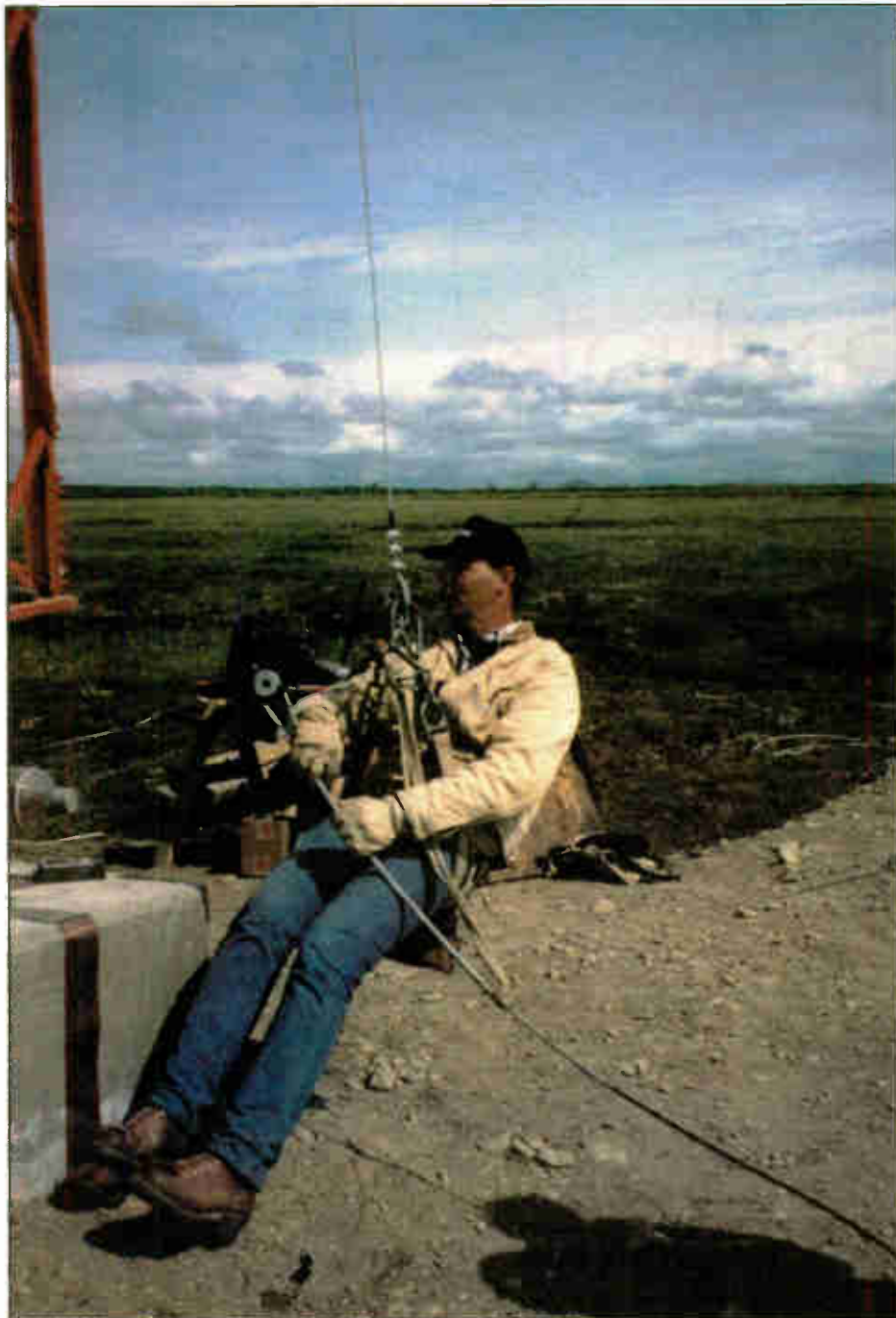
The tower erector prepares for ascent.
