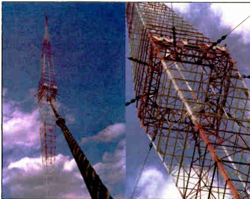
The antenna of WLW Cincinnati is a 747-foot Blaw-Knox diamond shaped vertical radiator, shown here in 1997. The middle of the tower was made wider (35 feet square) for additional structural strength. It has been in use since 1933. The bottom insulator supports a total stress load of 450 tons, including 135 tons of structure steel — 900,000 pounds.
