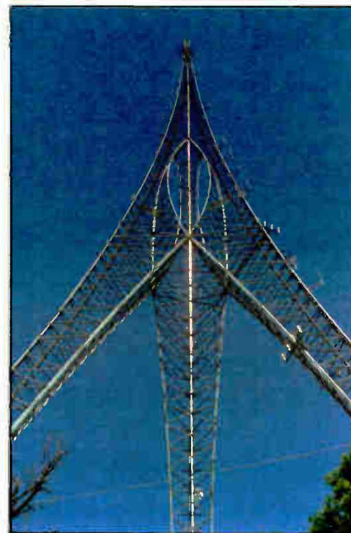
The Star Tower in Cincinnati, photographed in 2001. It was designed and constructed in 1991 by Landmark Tower Company of Ft. Worth, Texas. The upper sections were assembled using a helicopter.
