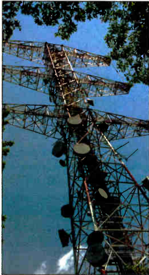
This is the 410-foot Armstrong Tower in Alpine, N.J., taken in 1988. It was built by Edwin Armstrong 50 years prior to that. From this tower, FM was first used for broadcasting. The structure also was used temporarily by New York FM and TV stations just after the World Trade Center attack.
