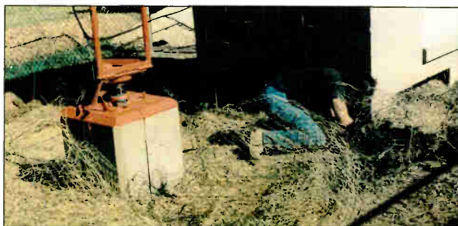
Fig. 2: Once the radials are identified, you can remove the old screen.
