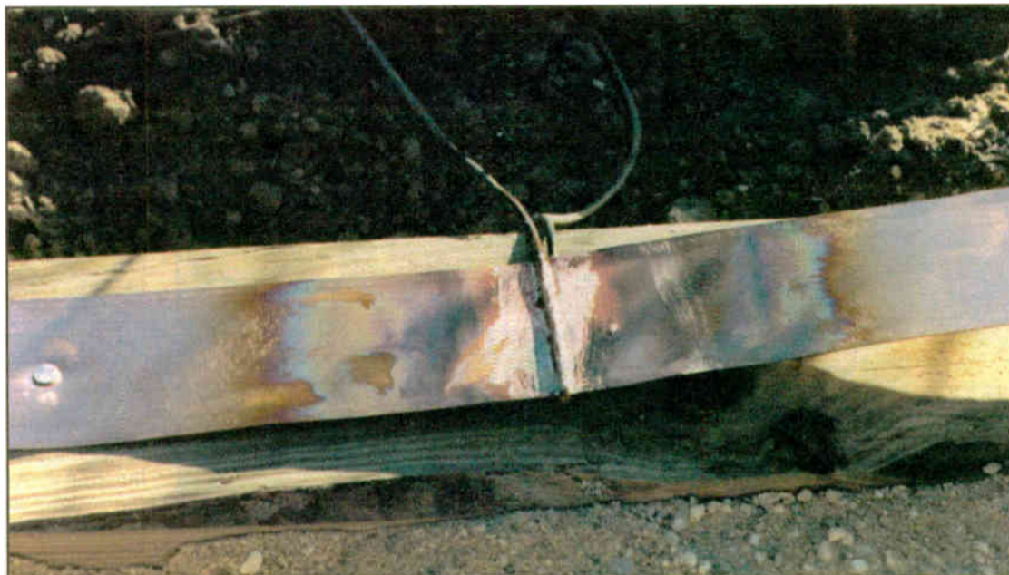
Fig. 7: The completed, soldered radial is shown.
