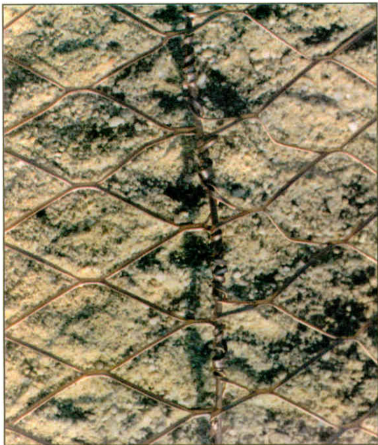
Fig. 4: The completed bonding of two pieces of ground screen is pictured.
