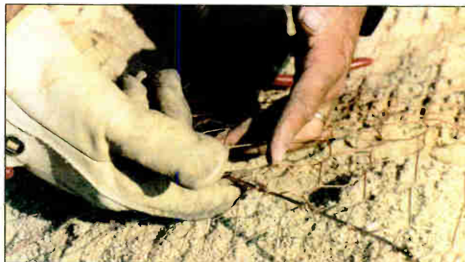
Fig. 3: Heavy leather gloves are helpful when piecing together the new ground screen.
