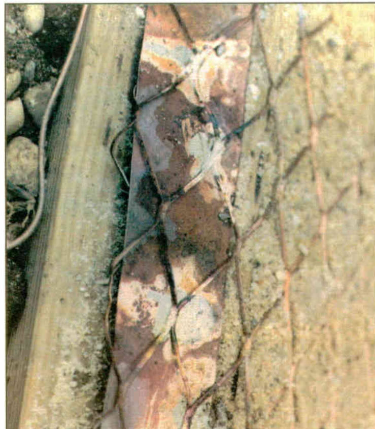
Fig. 5: The ground screen can be silver-soldered to the strap.
