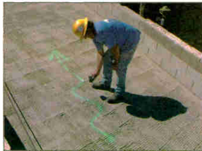
A tower worker in the KMEX driveway uses a meter to measure a 'hot spot' marked by the FCC with green paint.
