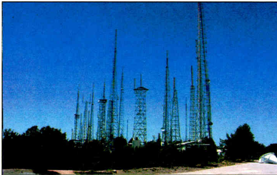
The Mt. Wilson antenna farm is home to more than two dozen FM and 20 TV transmission facilities.
