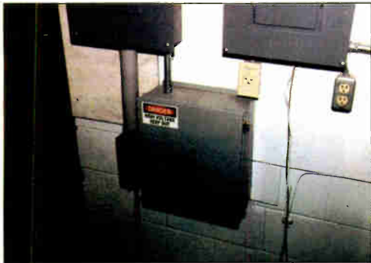
Fig. 1: Lights on this surge suppressor indicate the status of surge modules.
