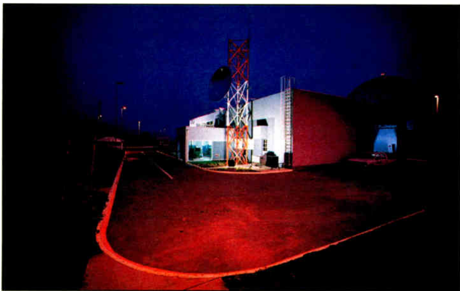
This publicity shot for Cummins reminds clients how much they have at stake should the power go off.
