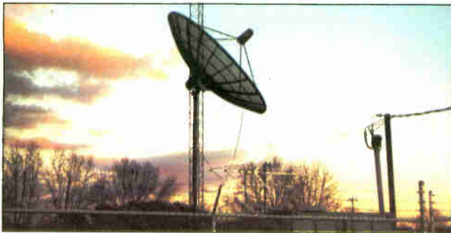
Fig. 2: Beautiful weather is a great excuse to check out what's happening on your building roof.
