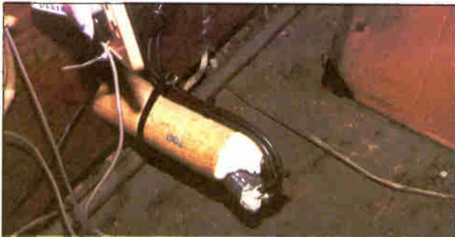
Fig. 3: Seal cable-entry pipes to keep out the elements.
