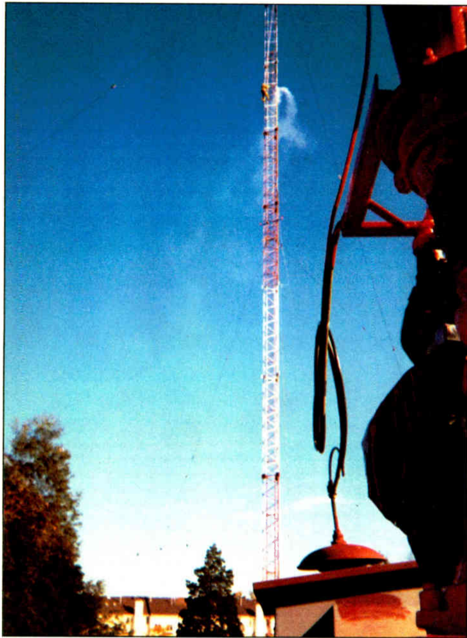
Fig. 4: The painting contractor is using compressed water to blast-clean the towers.
