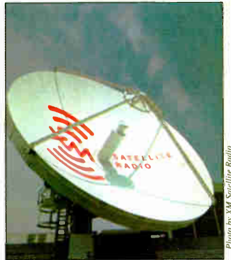
One of XM's two seven-meter uplink satellite dishes located at the facility
