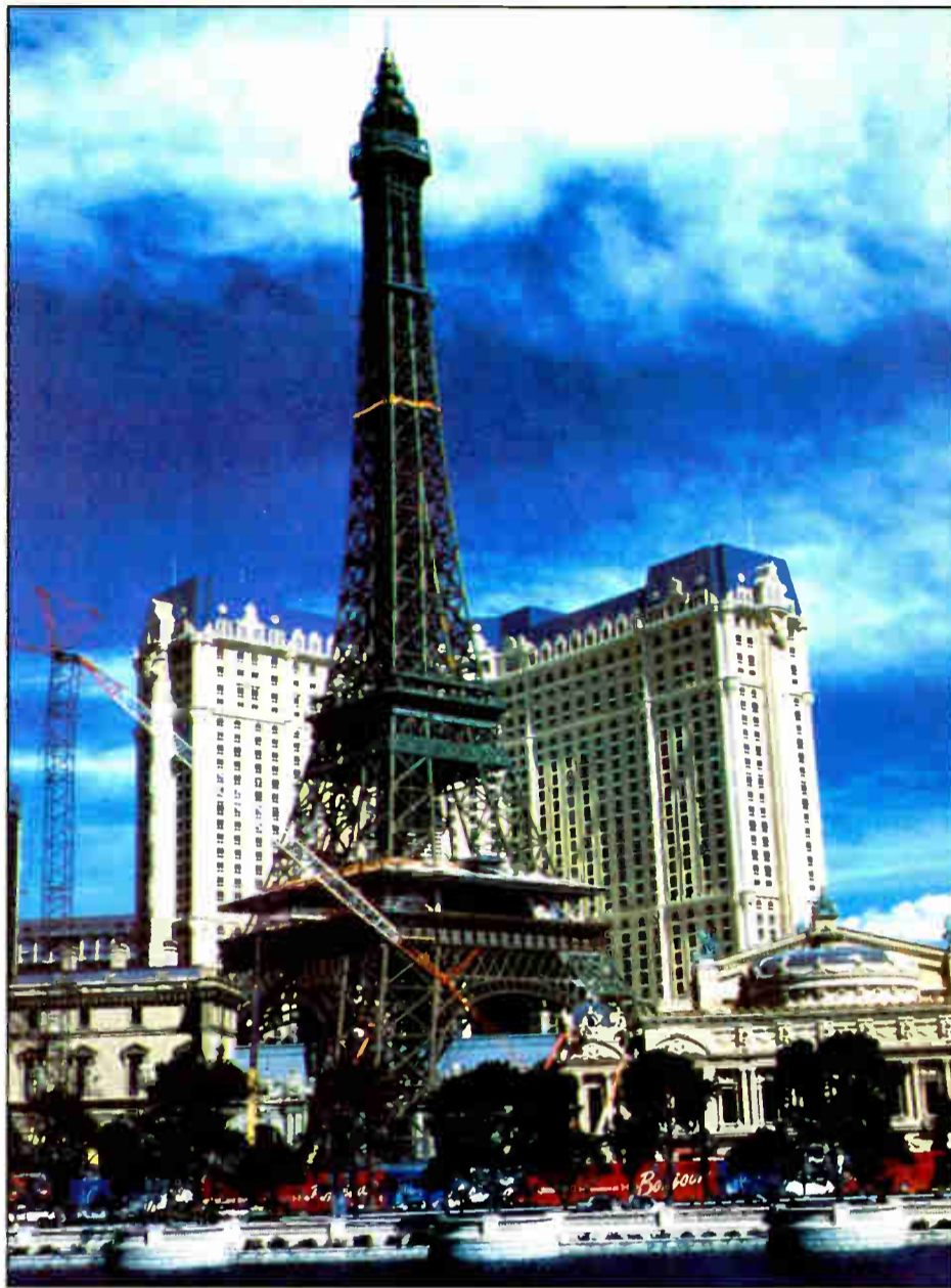
The Hotel Paris under construction
