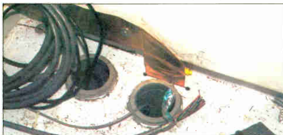
Fig. 3: Seal large-diameter conduits with a rag or steel wool
