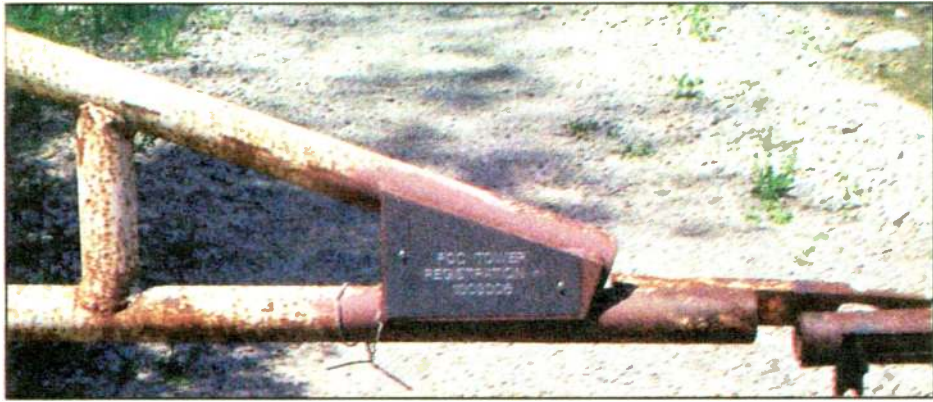
Tower registration numbers can be posted on the gate to the transmitter property.
