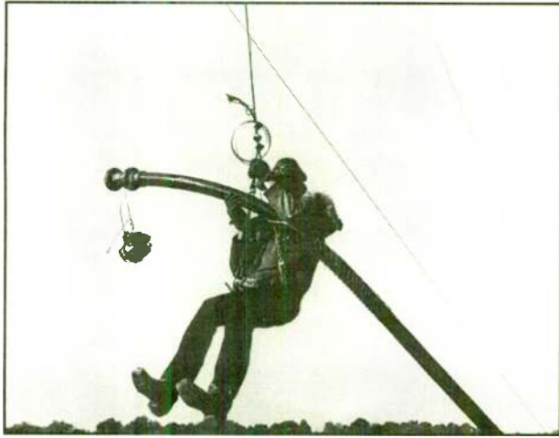
A tower worker prepares to install feedline.
