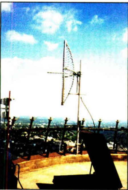
STL antenna atop Skylon Tower.
