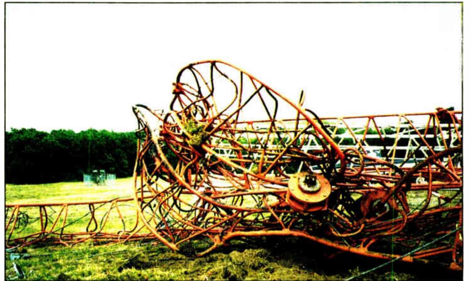
The 57-year old tower toppled in a few seconds.
