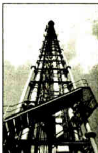
Coaxial Transmission Line
