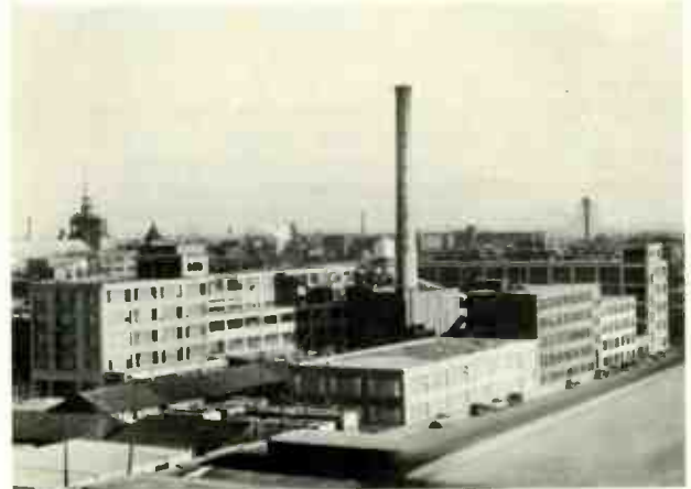
General View of the RCA Victor Company, Ltd.'s Plant in Montreal. The Engineering Products Division Occupies the New 2-story Building in the Foreground
