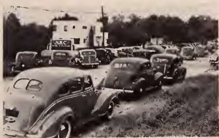
The NBC House of the Future on the day of its official opening.
