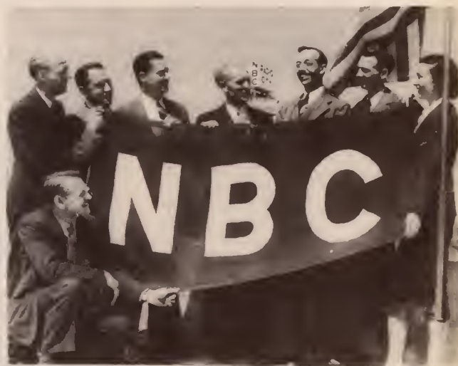
NBC engineers atop the last of the studio building roofs to be constructed in the Radio City of Hollywood which will be ready for occupancy in the Fall. Standing, left to right, Frank Figgins, studio engineer; J. J. Arnone, responsible for architectural details; R. F. Schuetz, in charge of the installation of broadcast and electrical equipment; Gordon Strang, job superintendent and engineer; O. B. Hanson, NBC vice president and chief engineer; Donald De Wolf, engineer in charge of NBC Hollywood, and Helen Welty, secretary to Mr. Strang. In front is Edward Nolen, assistant to Mr. Schuetz.
